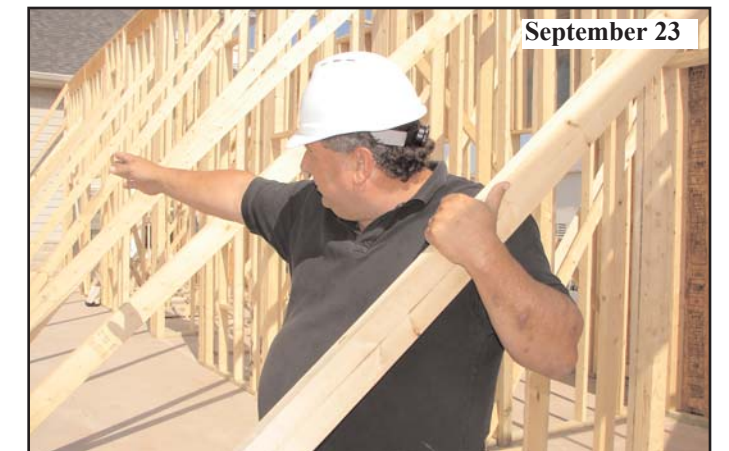
Winchester's Ron Keefer onsite and in charge.
